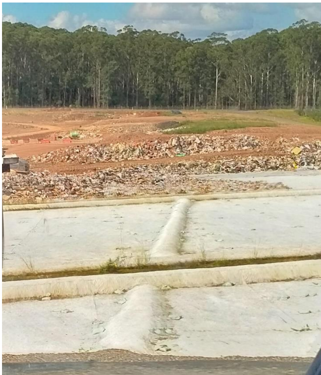
Image 1 shows part of the regeneration area with the white material laid down to filter the liquids. These are recycled or sent to the
