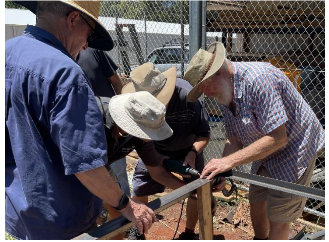
More teamwork. Dave drilling, with Howard, Greg and Will holding the metal steady. Metal a bit hot to hold!
